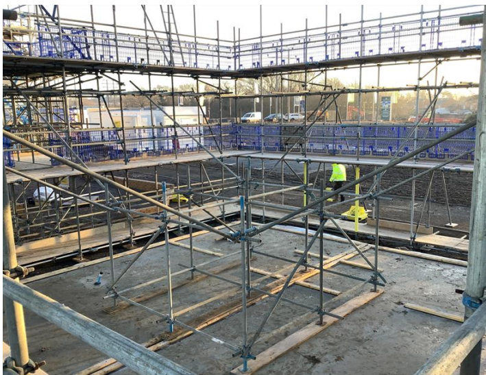
(Fig 2 example of inner buttress erected to prevent inward collapse)
