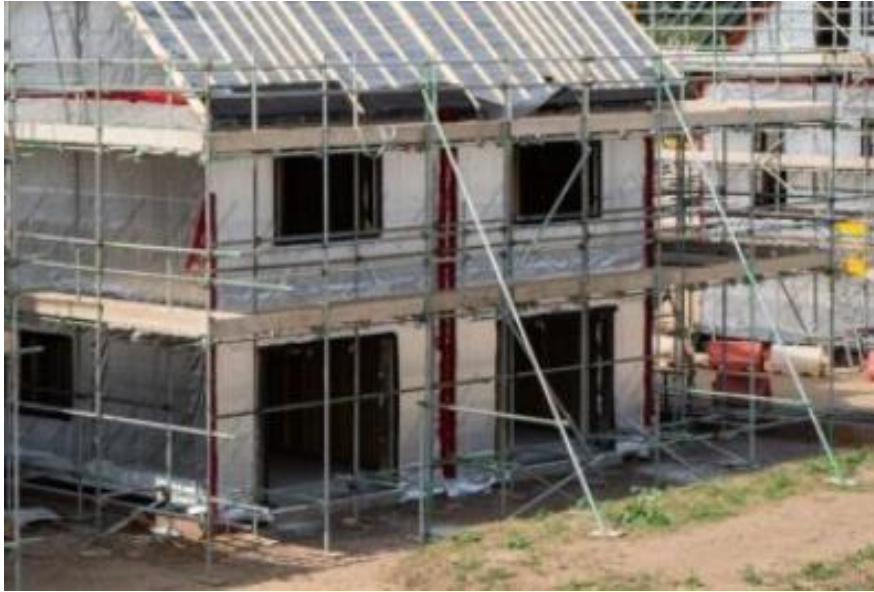
(Fig 1 example of external outriggers to provide stability to scaffold structure)
