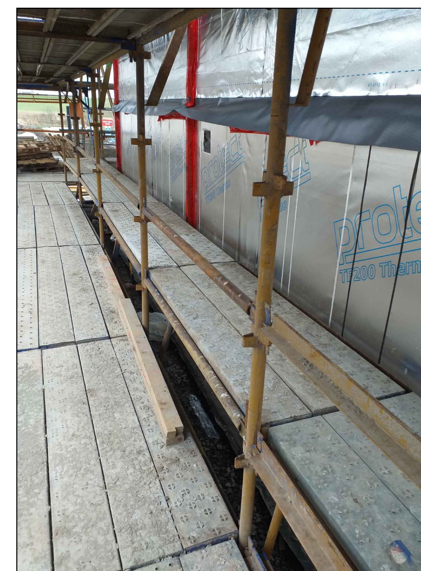
EXAMPLE IMAGE OF 1st HOP-UP/1st LIFT AT GROUND LEVEL.
