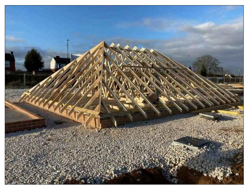
**GENERALLY SCAFFOLD BUILT AROUND ROOF CONSTRUCTED ON** GROUND. HOP-UPS TO BE LEFT OFF UNTIL ROOF LIFTED OUT ON DAY OF KIT ERECT.
