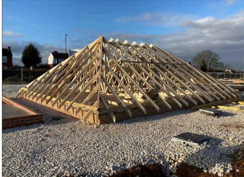
GENERALLY SCAFFOLD BUILT AROUND ROOF CONSTRUCTED ON GROUND. HOP-UPS TO BE LEFT OFF UNTIL ROOF LIFTED OUT ON DAY OF KIT ERECT.
